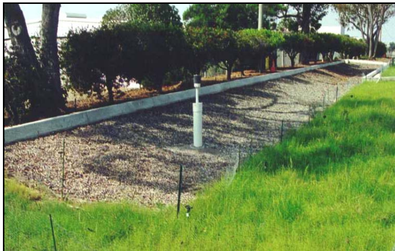
Figure 6-3: Typical Infiltration Trench (CASQA, 2004)
