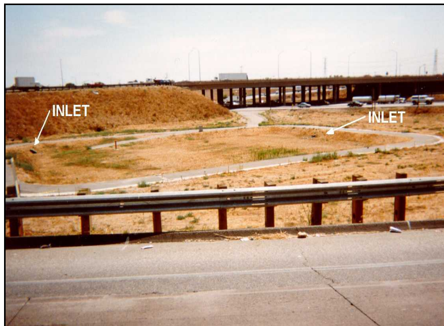
Figure 6-5: Typical Infiltration Basin (CASQA, 2004)
