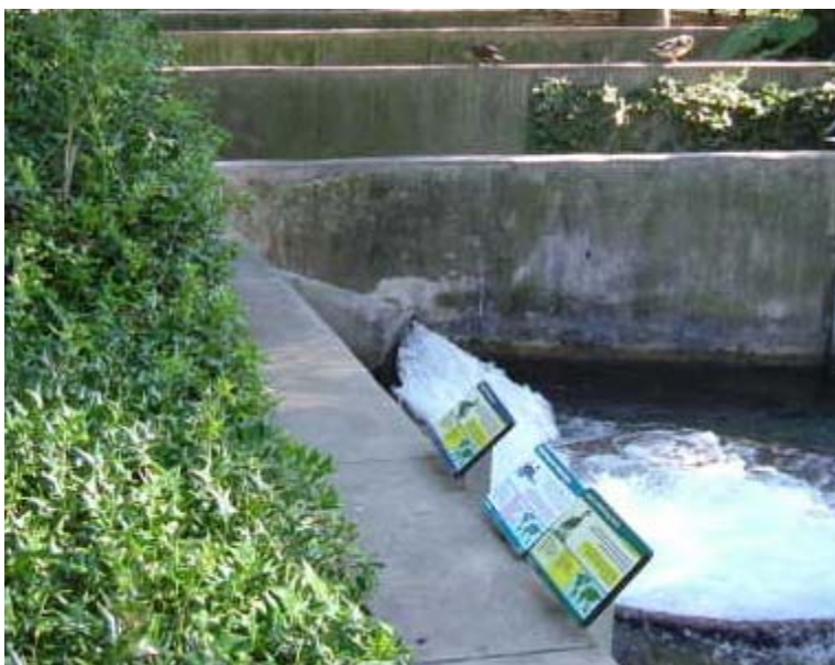
Figure 3-20: Discharge from Zoo Well House
