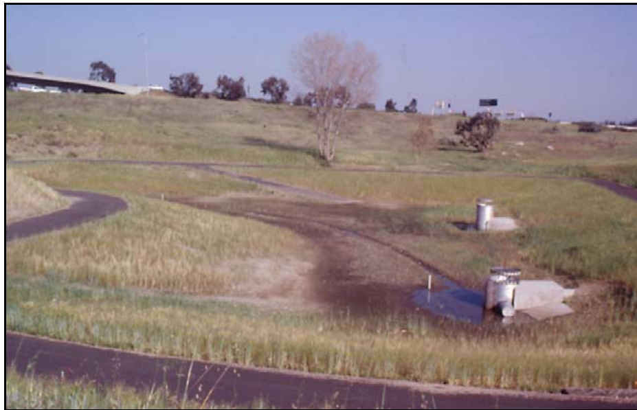
Figure 6-11: Typical Extended Detention Basin (CASQA, 2004)
