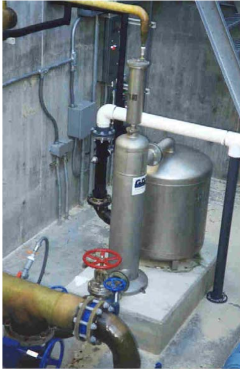
Figure 5-5: Ozone Side stream Contactor and Degasser
