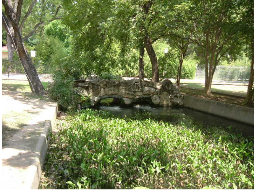
Figure 3-8: Primary Outfall Channel just outside of Zoo
