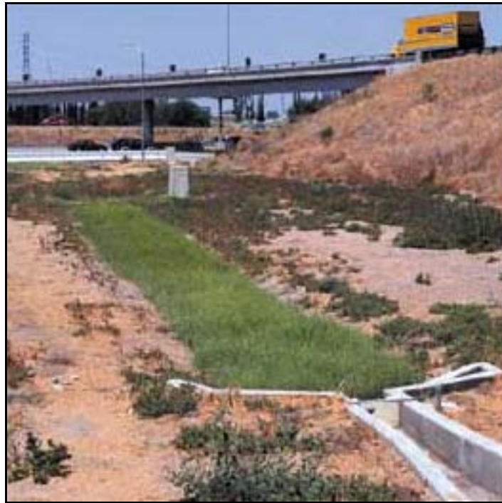
Figure 6-13: Typical Swale (CASQA, 2004)
