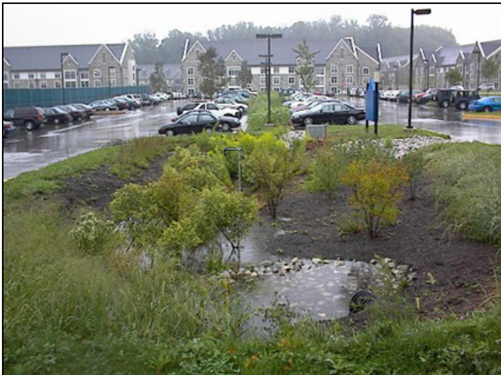
Figure 6-14: Typical Bioretention Basin (CASQA, 2004)
